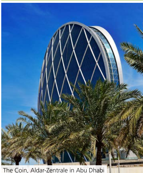
The Coin, Aldar-Zentrale in Abu Dhabi
